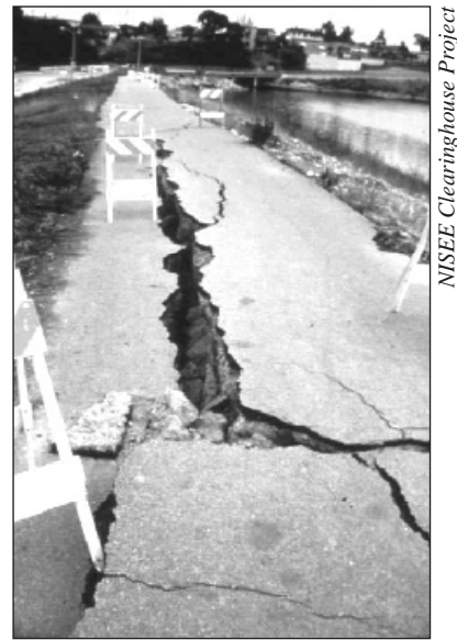
Figure 35 - Lateral Spreading, Loma Prieta Earthquake, October 17, 1989. Lateral spreading damaged levee road along the San Lorenzo River.
