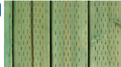
Treated wood often has holes where treatment was injected.
