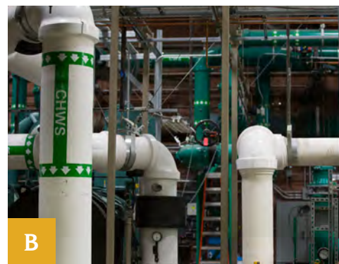
A: The future campus energy plant will be integrated with the design of a new building. (Source: SJSU)
